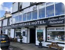
9. Harbour View Restaurant (The Islay Frigate)
